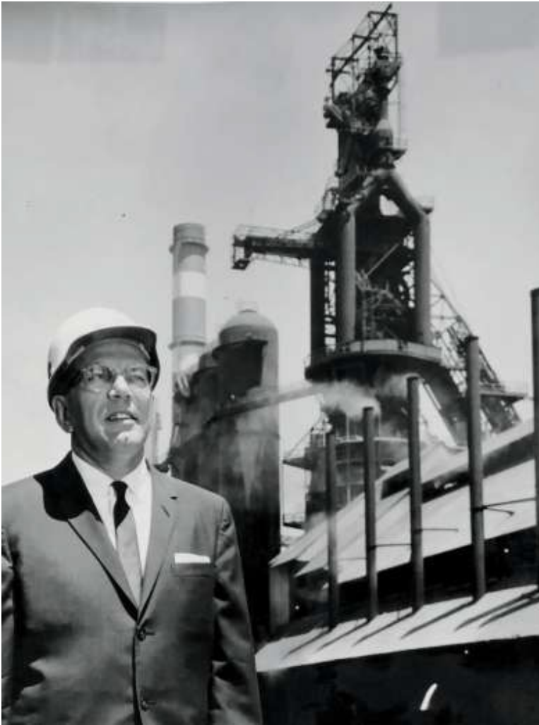
Along one of the three blast furnaces at Geneva Works
